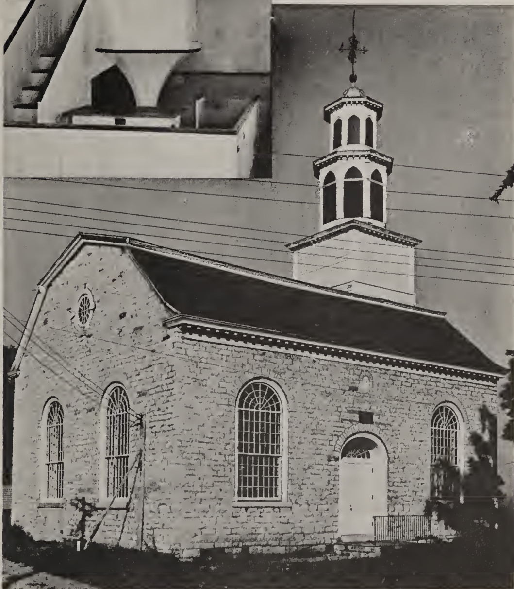
THE OLD PALATINE CHURCH (SHRINE) BEFORE THE RESTORATION OF 1952 WAS COMPLETED
